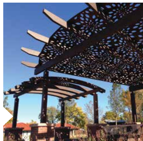
Pattern: Lemon Drop [ contemporary ] Project: Sloan's Lake Pavillion (Denver, CO) Material: 1/4" aluminum Support: 32" on-center Designer: DHM Design
